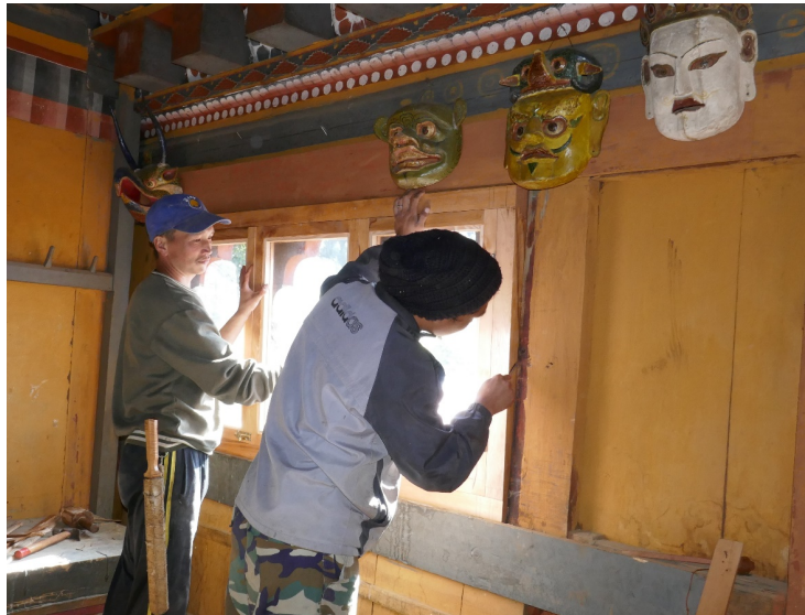
Fixing a window frame
